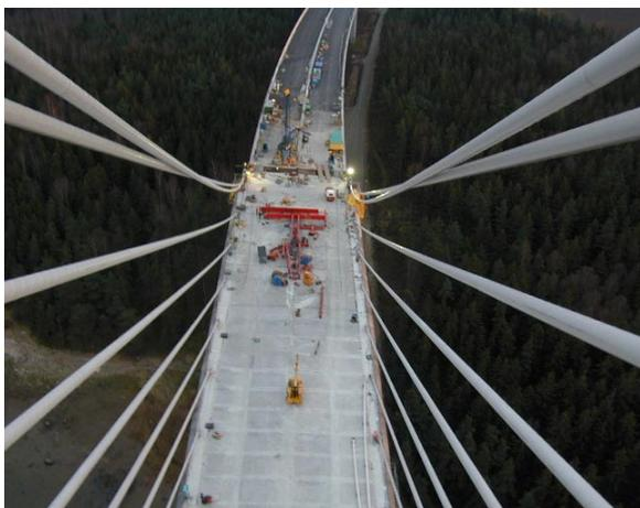
Fig. 1 *Visible sagging of long stay cables highly influence forces in the stay cable*
