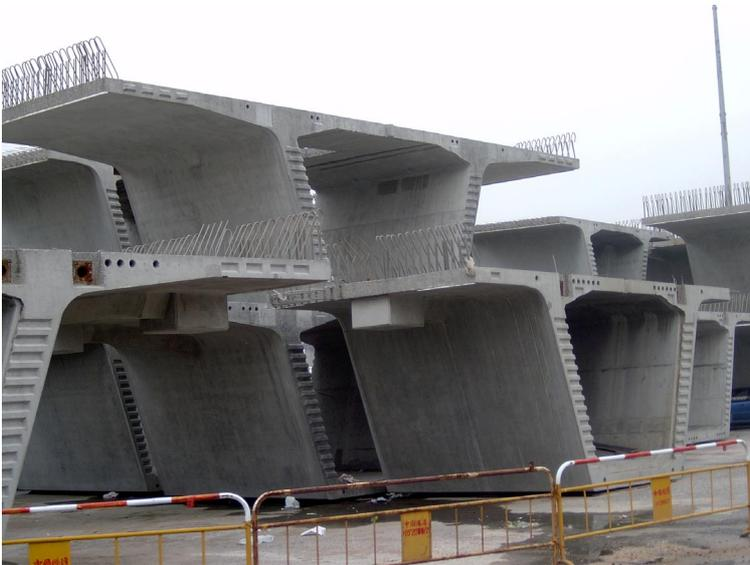
Fig. 4 Segments waiting for erection
