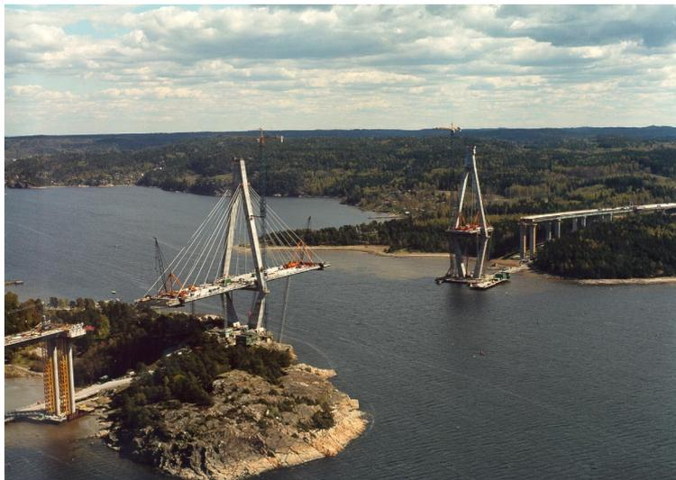
Fig. 5 Typical construction stage for stayed cable bridge
